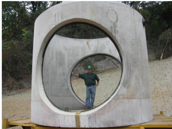
The 72" diameter reinforced concrete pipe was produced with rubber gasket joints and requires field testing in accordance with ASTM C1103. The 126" diameter precast manholes were produced with ALOK pipe connections to receive the 72" diameter concrete pipe. Construction is expected to continue through most of 2011.
