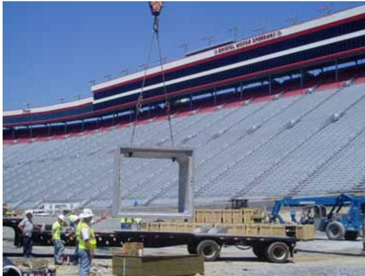
A section of 9' x 8' precast concrete box culvert being unloaded at the project site at Bristol Motor Speedway.
