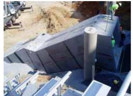
Precast box culvert being installed as a pedestrian tunnel with grade changes and varying fill heights.
