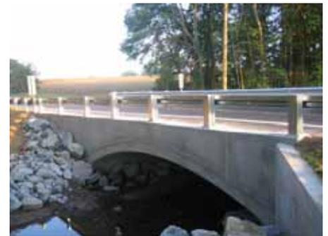
Hanson Pipe and Precast produces its Hanson Arch in 12-foot to 48-foot spans. Some of Hanson's arches are used as small bridges and some as arch culverts.
