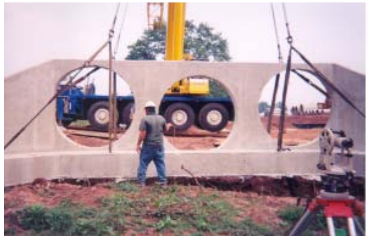
Frederick Precast helped create the biggest endcaps in Maryland.
