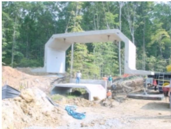
*The OmegaSpan is a three-sided bridge structure that requires no cast-in-place footings.*
