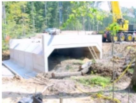
*The OmegaSpan is quick to set and lasts longer than the corrugated metal arch.*
